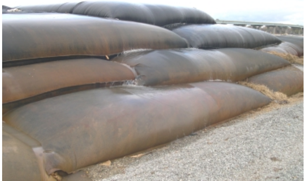
Geotube® containers stacked in a dredging operation at Fox River. Geotube® dewatering containers can be layered like this to increase dewatering volume for the space allotted. For a large project, this can be critical.
