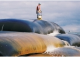
An operator using a mechanical vibrator to break up caking inside the unit and to make dewatering even faster. Note water flowing from the units.
